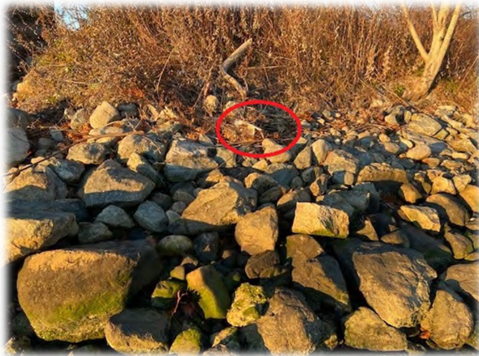
Existing 4" PVC Discharge to be Replaced Upslope (CB-E Watershed)
