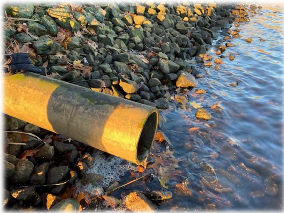
Existing 10" PVC Discharge to be Replaced Upslope (North Watershed)
