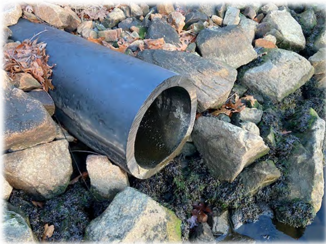
Existing 20" PE Discharge to be Reused (Middle Watershed)
