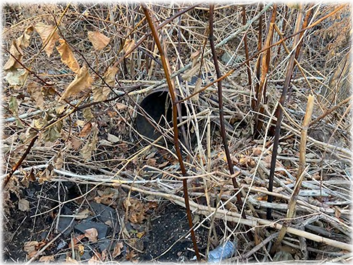
Existing 24" CI Drainage Discharge from 133 Depot Road (West Watershed)
