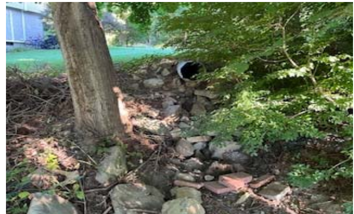
Culvert from Catch bason from Cedar Lane
