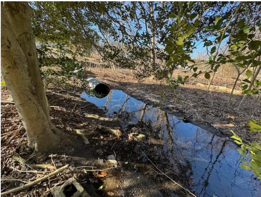
Photo 2: Sharp Hill drainage discharge point. Note sediment buildup.
