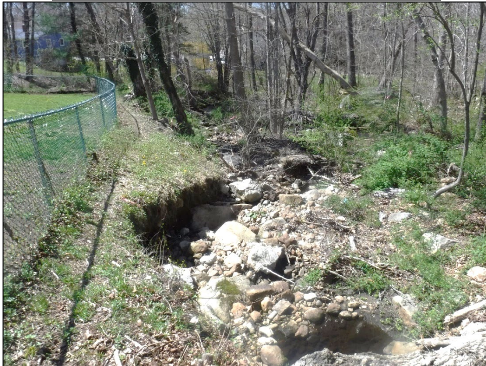
Photo 4 – Erosion of Channel Embankment (Looking Downstream)
