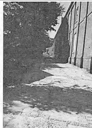
Backfilled and compacted excavation area to the west of the site building.
