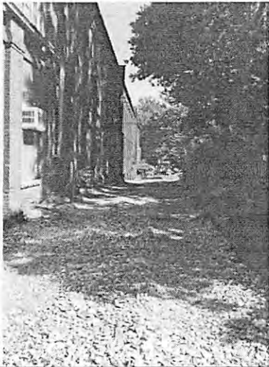
Backfilled processed stone prior to paving.
