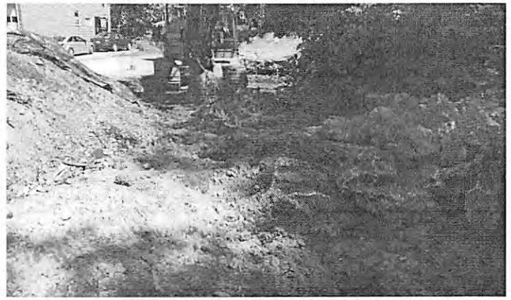
Material segregation in the stockpile area.
