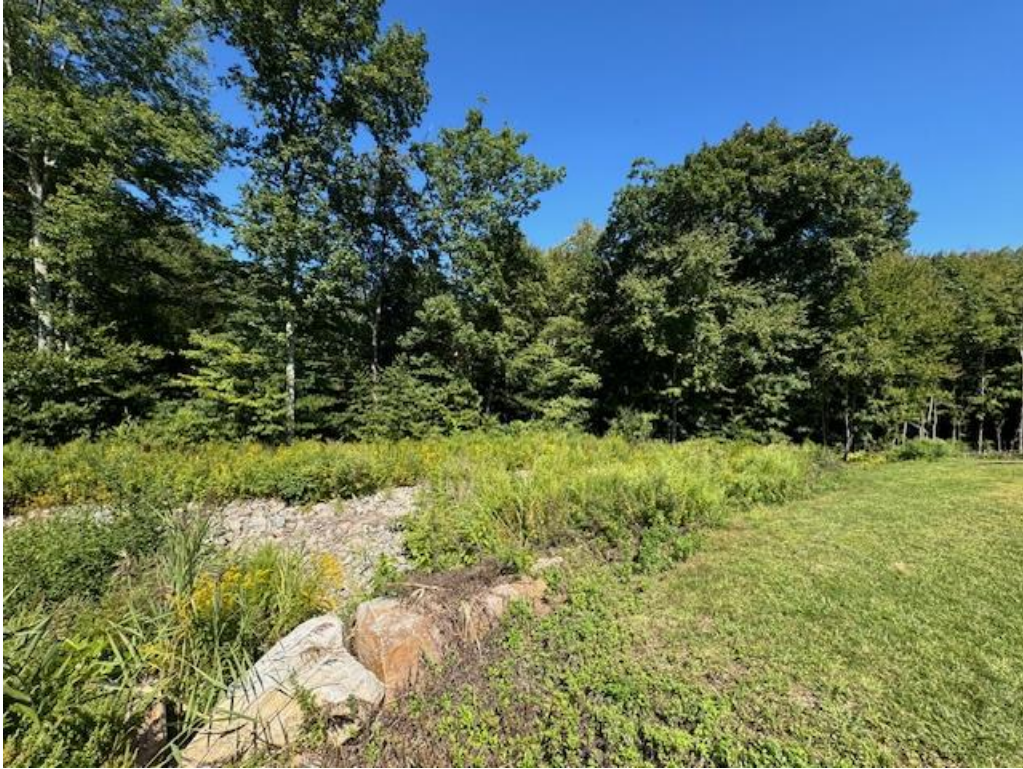
Photo 5: General conditions at end of Carol Drive and example of the man-made stormwater drainage features that have been somewhat recently installed.
