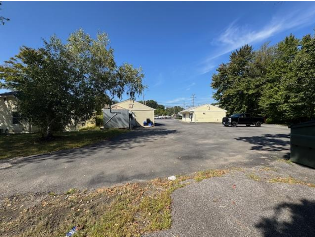
Photo 5: General developed conditions on the western half of the site, these structures will be demolished and removed from the site.
