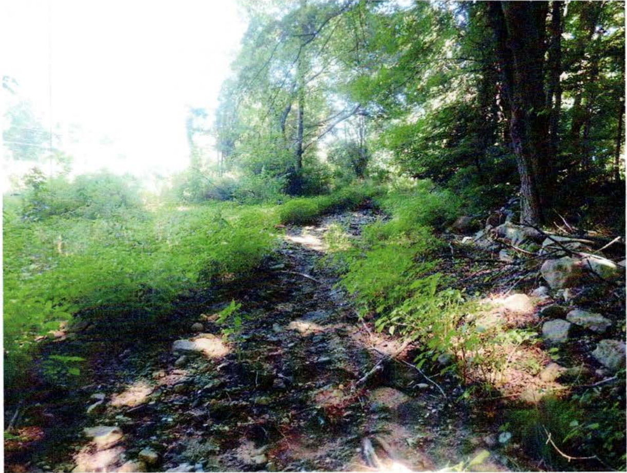
Photograph 4 – Surface erosion/shallow channel downstream (taken looking upstream toward transect location)
