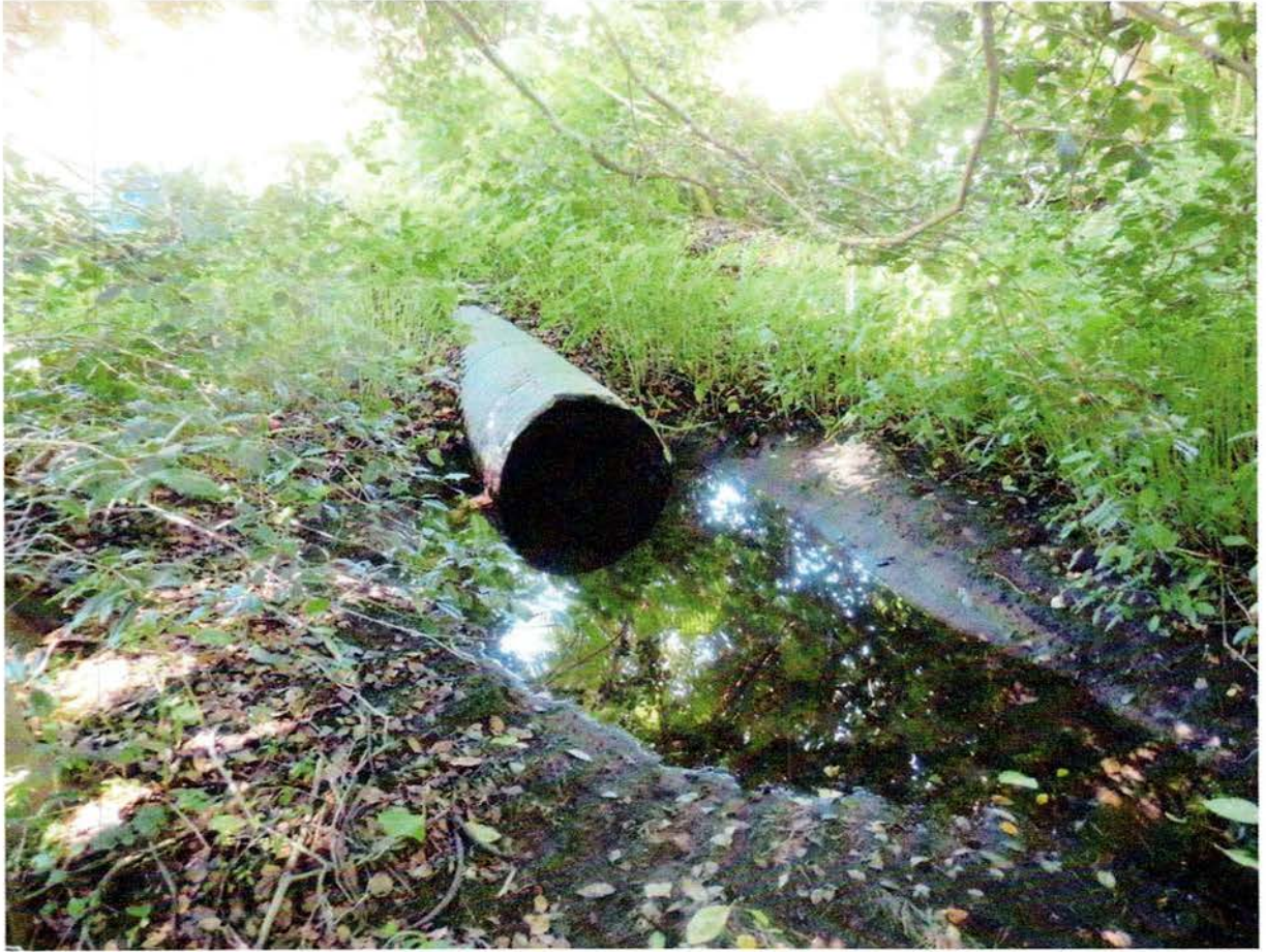
Photograph 3 – Wetland at 36-inch culvert outfall
