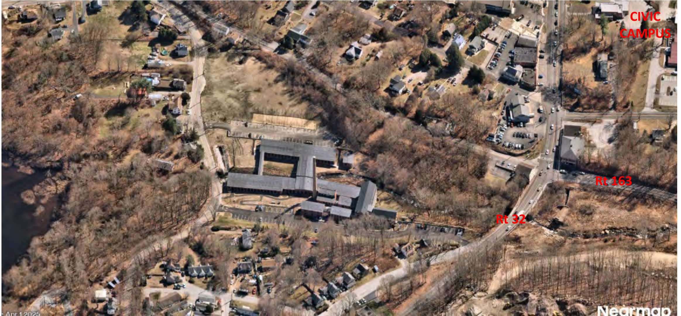
Exhibit 7: Oxoboxo Lofts and Village Apartments
