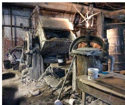
Clockwise from above: Equipment left on-site when the Boyertown Burial Casket Company factory closed in 1988; an aerial view of the three buildings that became The Willows; the foyer with exposed brick and loft space. Below, Pattie E.B. Guttenplan, AICP, RLA, deputy director for the Montgomery County Planning Commission, credited part of the success to working with developers familiar with building low-income housing.
