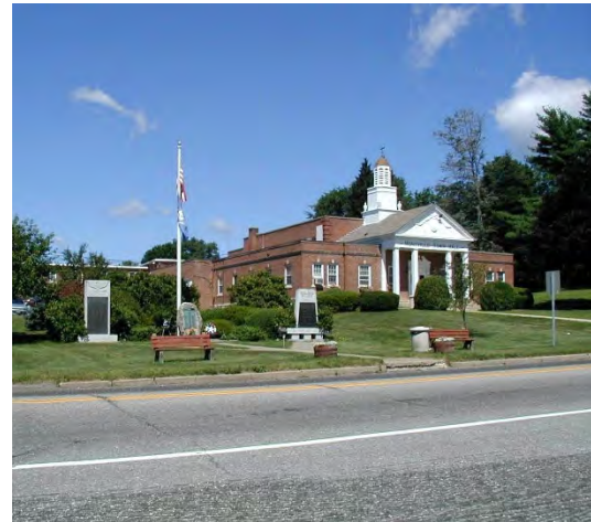
Town Hall Annex
