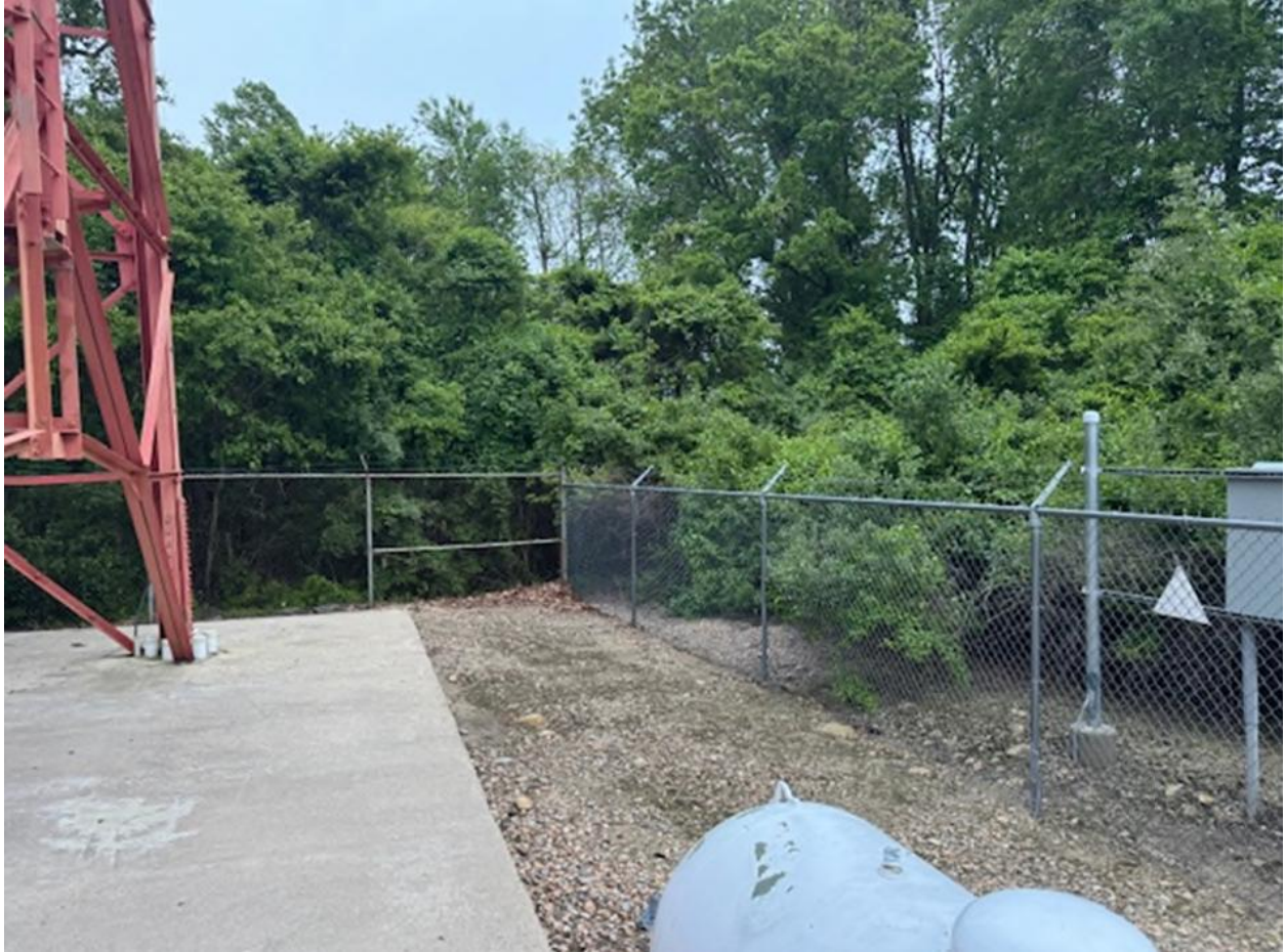
Figure 5 – Existing Facility Fence to be Modified
